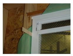
sill. A minimum 1/4" gap should be maintained between the sill of the window and the construction sill of the wall to allow for proper weeping and drainage from the window when shimming.
