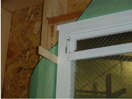
Once the window is centered and properly shimmed the interior sill angle can be installed. The long leg of the angle generally attaches to the wall. After the sill is screwed down the two remaining jamb angles can be trimmed to the dimension measured between the top of the sill angle and the bottom of the interior leg of the headcap. The longer leg of the interior jamb angles generally goes to the wall and can now be affixed into place.
