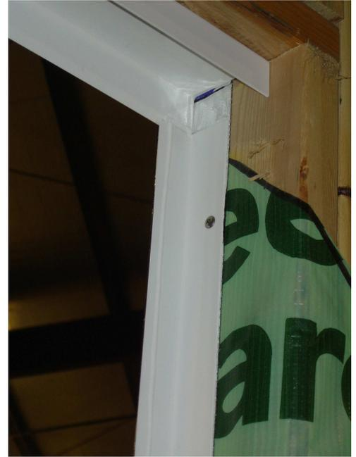
The interior trim should be screwed to the window at intervals of no less than 2" from each component end and 24" on center thereafter.
